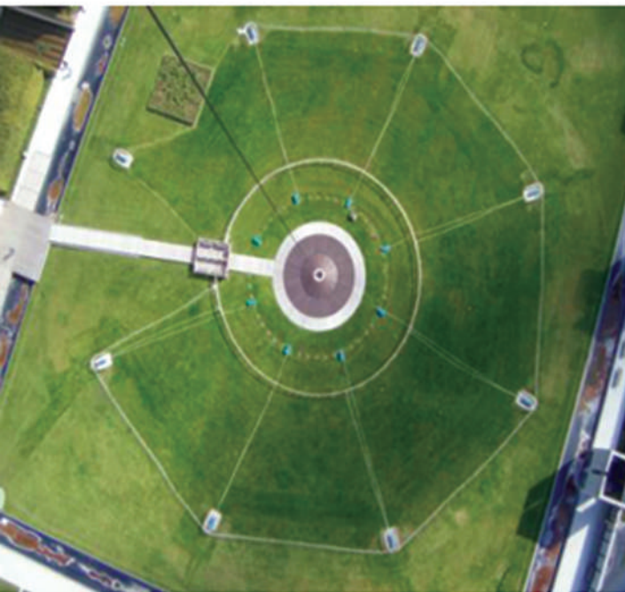
Paris – installation on ground
